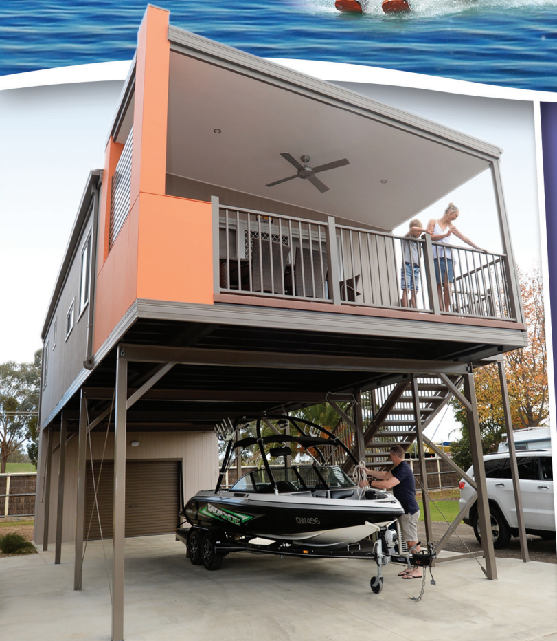
One of two new high-rise apartments at our Ski Club Holiday Park
